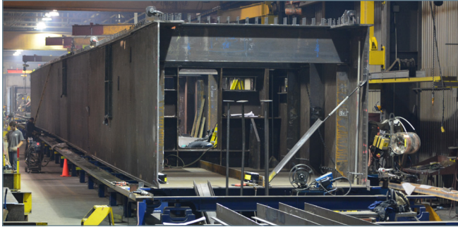
Steel component of the new Champlain Bridge • Montreal, Canada
