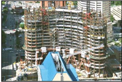
Encana Tower (The Bow Project) Calgary, Alberta
