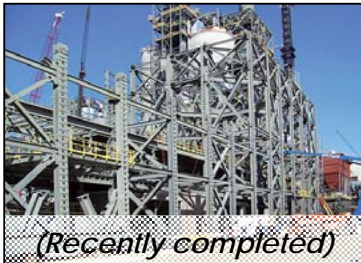
Holcim Cement Plant Ste. Genevieve, Missouri
